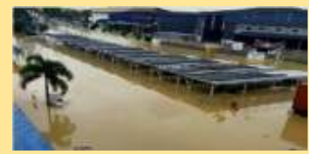
Flood incident in December 2021
