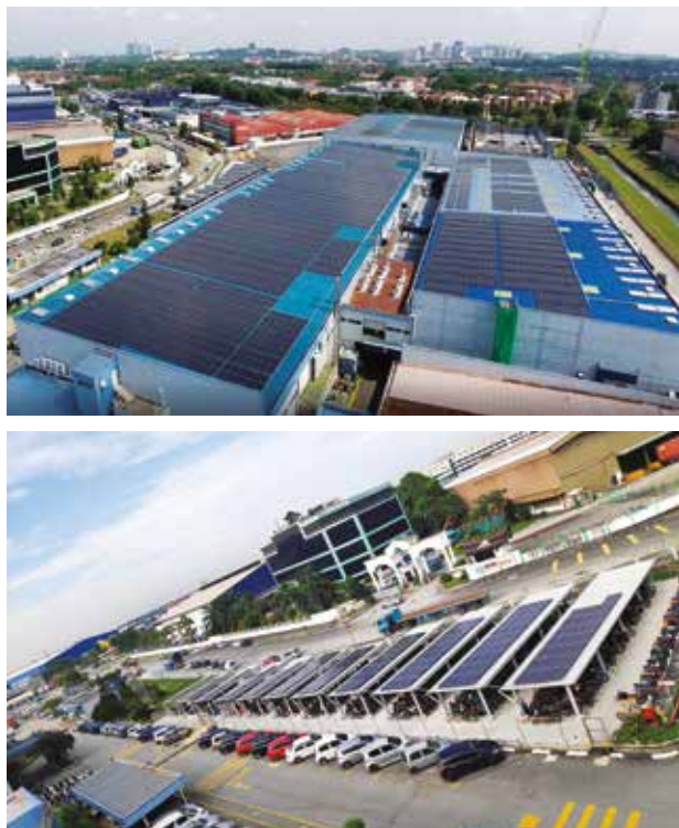
Solar Panels installed at SA2 Plant
